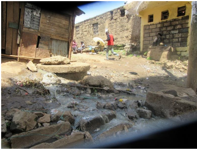
Photo 9: Burst sewer lines.
